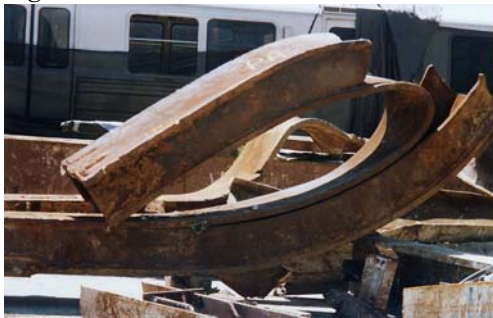
Figure 3. Distorted WTC Steel Beam
